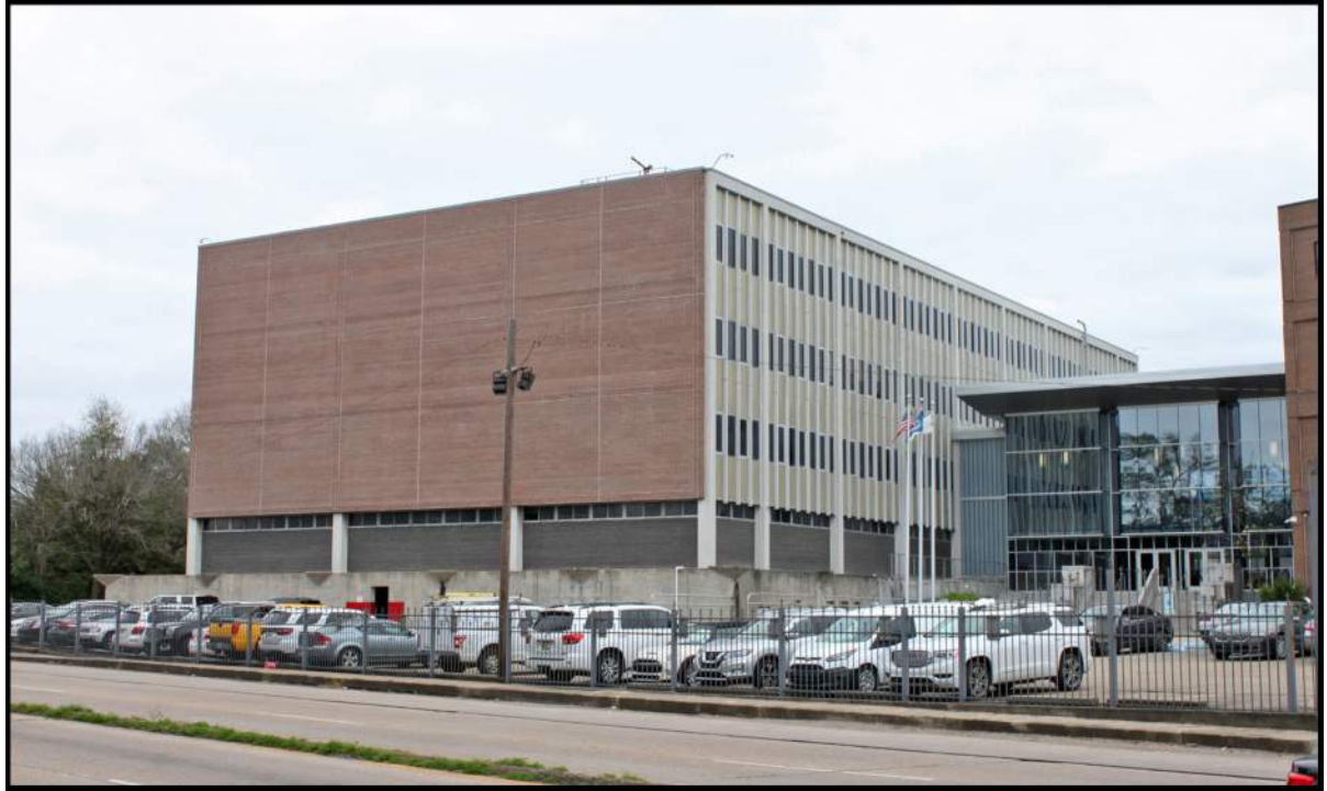
Figure 4-21. The Louisiana Workforce Commission building was designed by LeBlanc & Deen. View is to the northeast.
