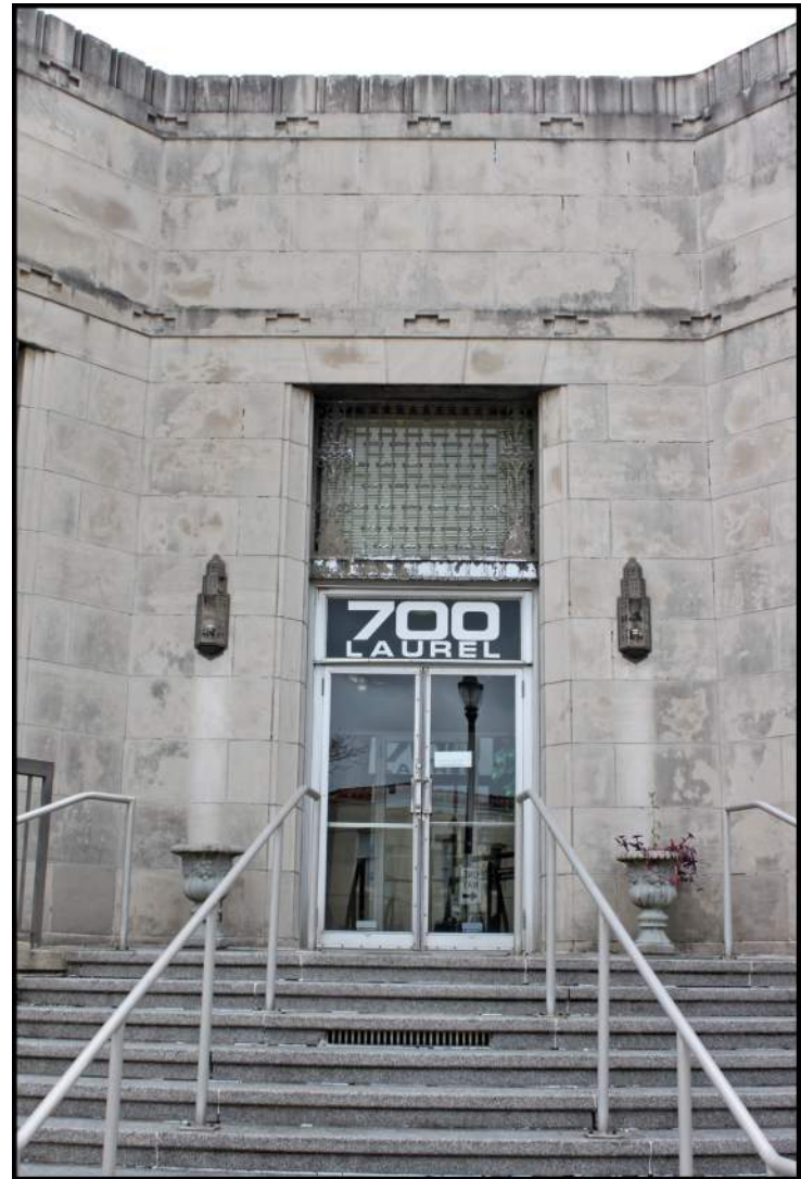
Figure 4-9. The original transom, door surrounds and Art Deco sconces remain at the entrance to the building.
