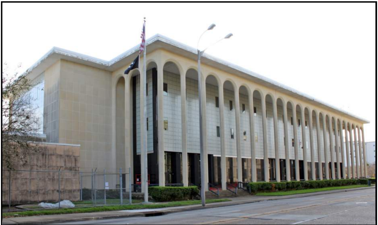
Figure 4-20. Recent updates to the building include covering the existing windows with opaque glass. View is to the southwest.
