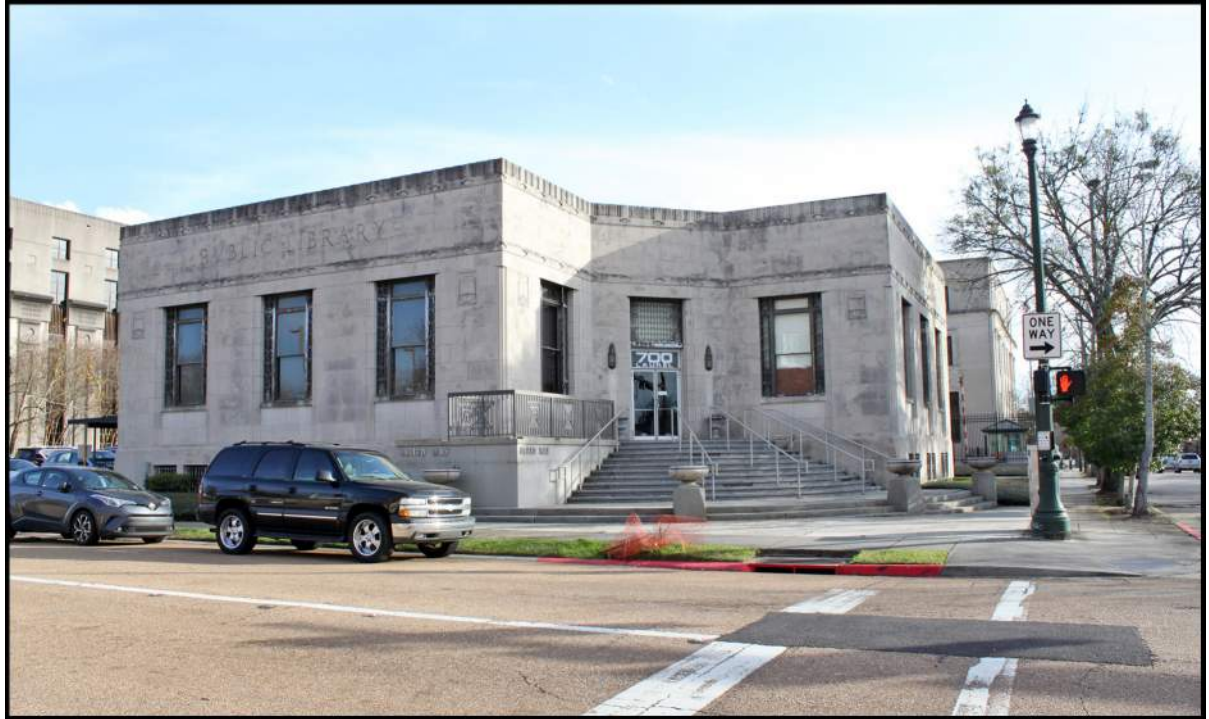
Figure 4-6. The Old Public Library was built in the Art Deco style. View is to the southeast.
