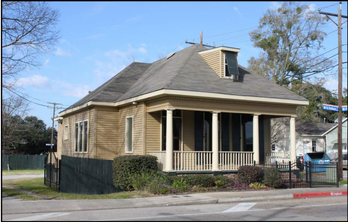
Figure 4-4. Structure 17-00278 is the only Beauregard Town NRHD central-hall house located within the APE. View is to the northwest.
