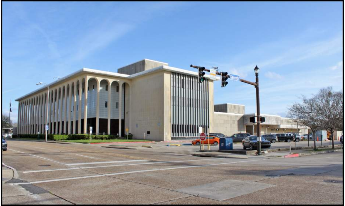
Figure 4-19. The U.S. Post Office at 750 Florida Street is an excellent example of the New Formalism sub-style. View is to the southeast.
