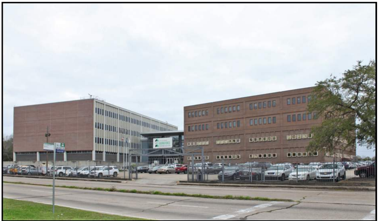
Figure 4-22. A glass-walled foyer was added recently to the building to attach it to the 1980s building to the south.
