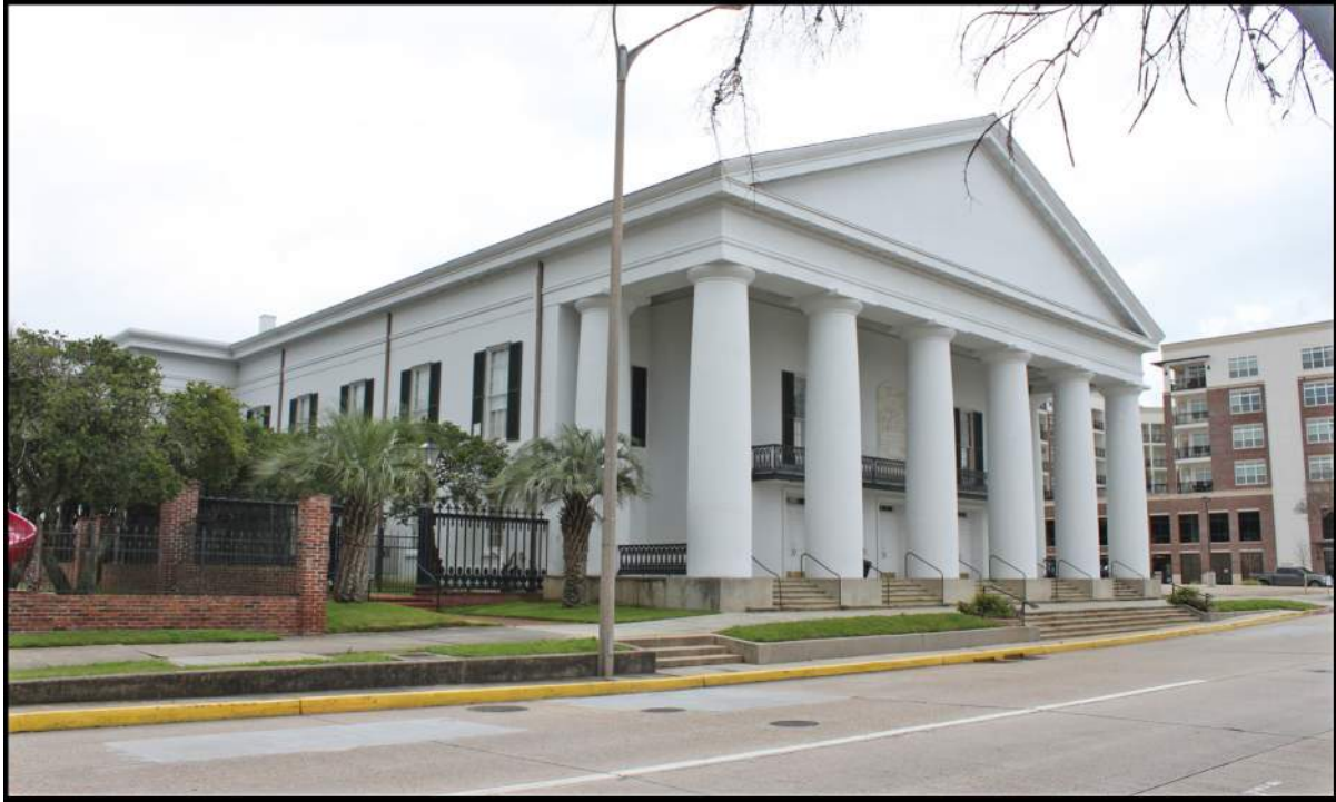
Figure 4-16. The cupola shown in Figure 4-15 is no longer extant. View is to the northeast.
