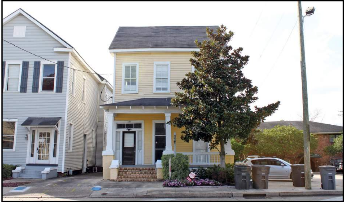
Figure 4-2. Structure 17-00277 is the only Beaugard Town NRHD bungalow located within the APE. View is to the west.
